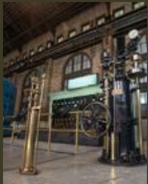
Niagara Parks Power Station
